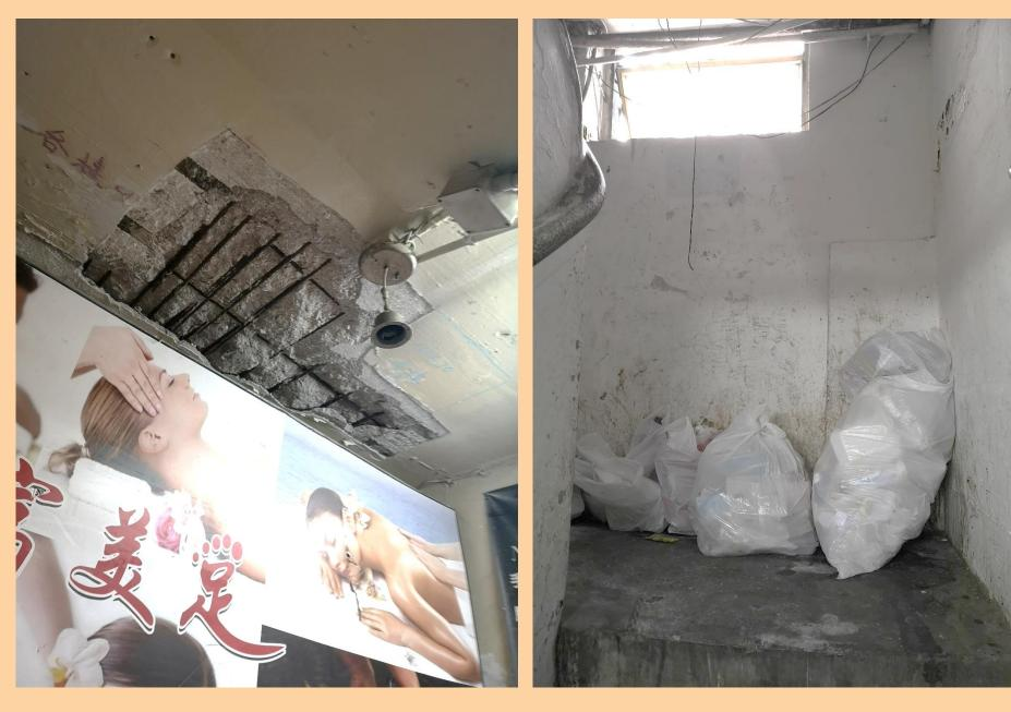
Figure 1: Exposed reinforcement on ceiling
