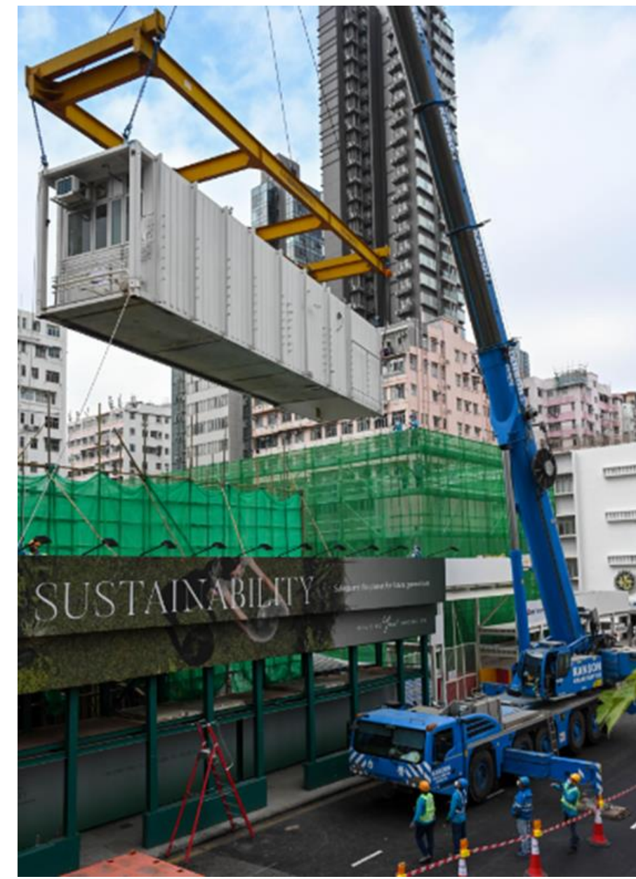
Fig 2: Relocatable MiC module in Nam Cheong 220
